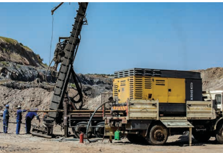
A blasthole rig being established.
