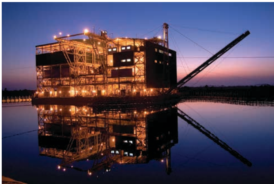
One of the major projects for Fluor was Rio Tinto’s Ilmenite mine’s wet plant in Madagascar.
