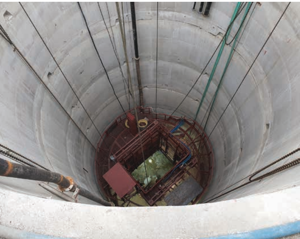
Pre-sink stage view from bank elevation.
