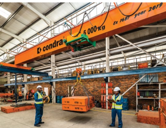
The 13 cranes already installed were designed and manufactured in Johannesburg by BB's parent company, Condra.
