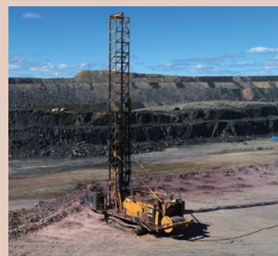
A Drill-to-Mill strategy is expected to be deployed based on a series of tightly integrated systems, driven by Cat MineStar solutions.
