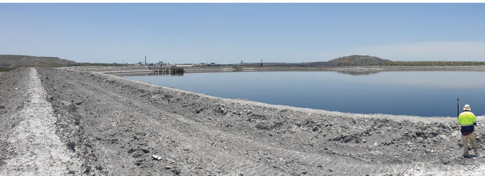
The gypsum stacks at the Phalaborwa Rare Earths project.
