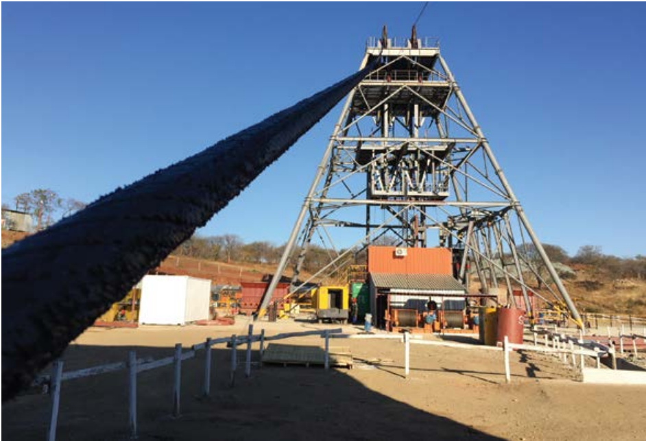
Solar plant powers Caledonia Mining's Blanket Mine.
