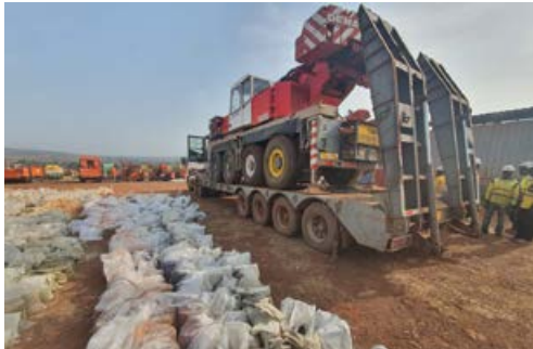
Kouroussa Gold Mine construction moves apace.
