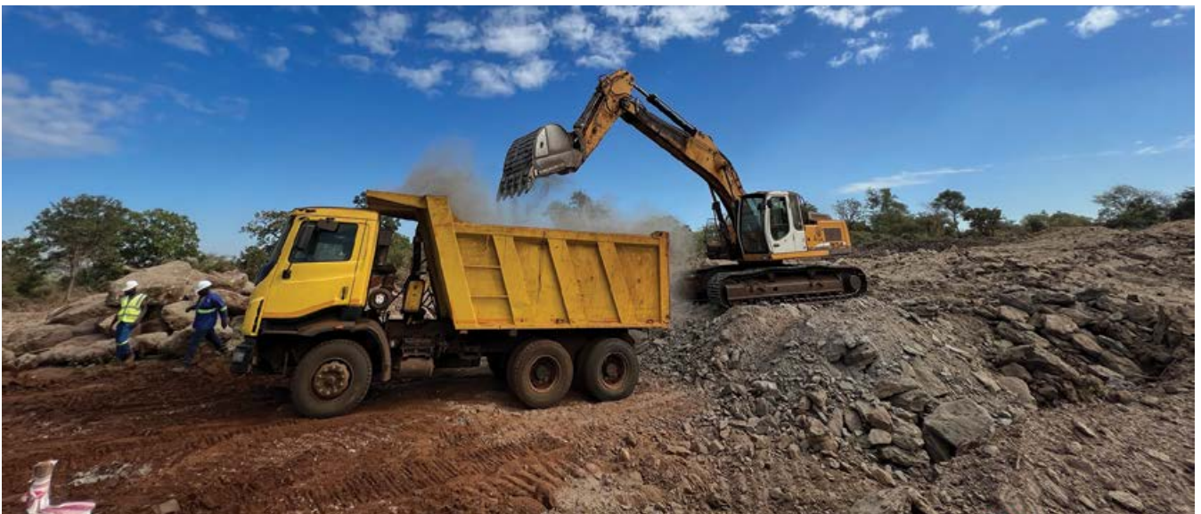
Loading and hauling underway at the Lindi Jumbo project.
