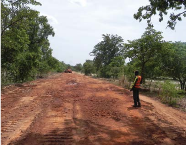
Road construction underway.
