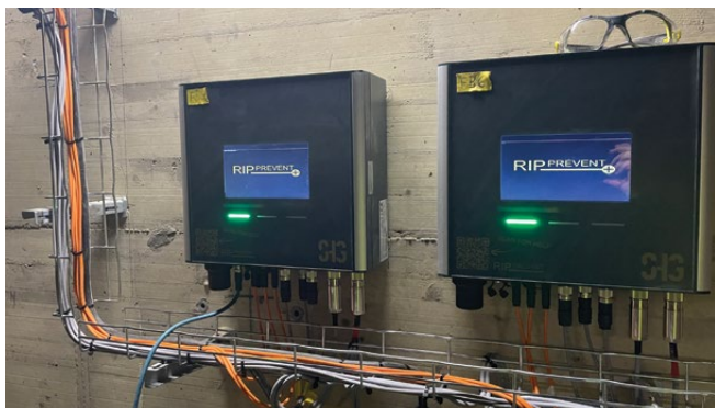
Tru-Trac's Rip Prevent+ monitoring system uses AI to detect anomalies before they escalate, enhancing safety and reliability.
