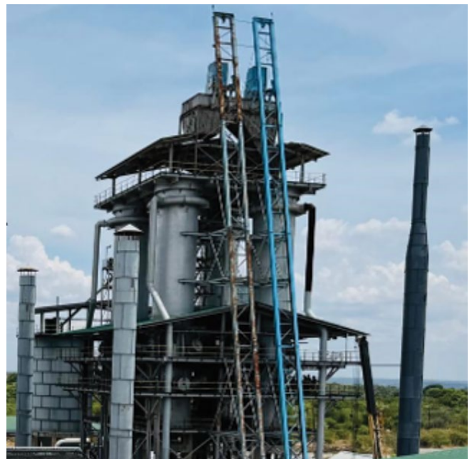
View of kiln 1, the first fully operational kiln at the Limeco Plant.
