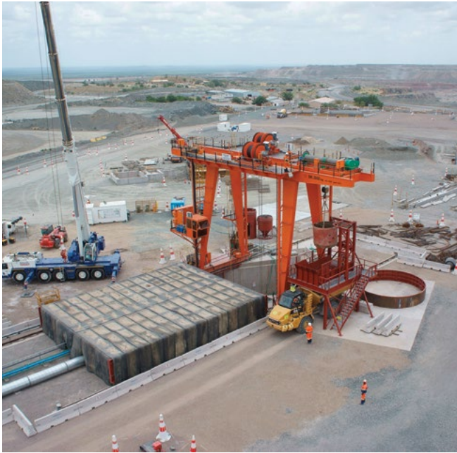
The pre-sink gantry arrangement at Venetia Mine with a blast cover and kibble tipping arrangement.
