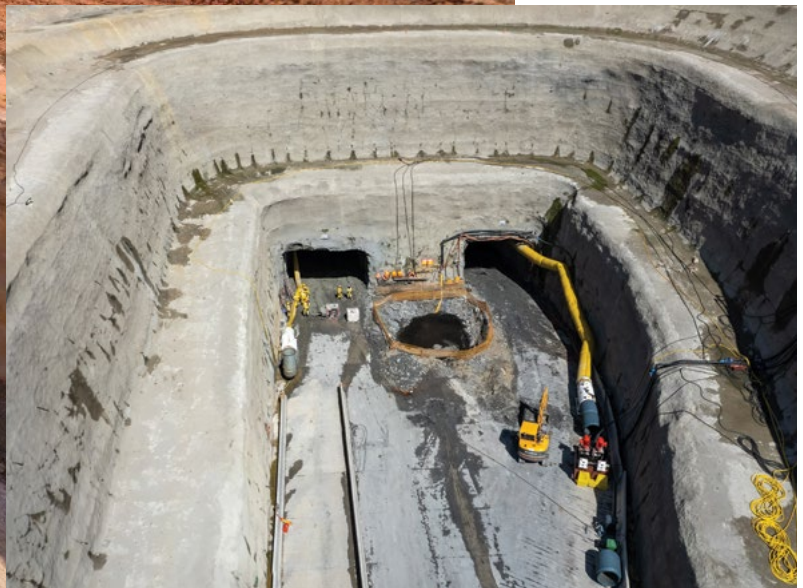
The box cut at Matla Mine is captured here, forming the critical entry point for developing new underground access to coal reserves.
