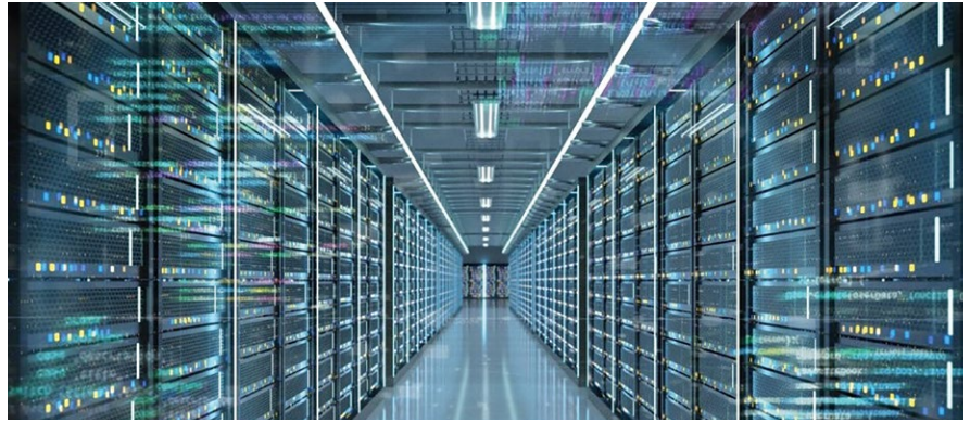
Rapid growth in AI data centres is driving demand for resilient, high-capacity energy infrastructure.
