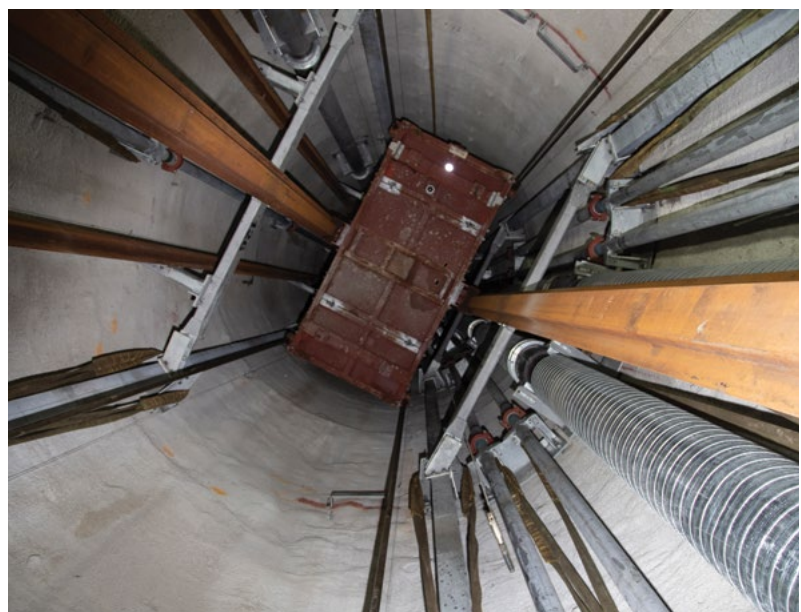
Zondereinde Western Expansion Project 3 Shaft men and material shaft.
