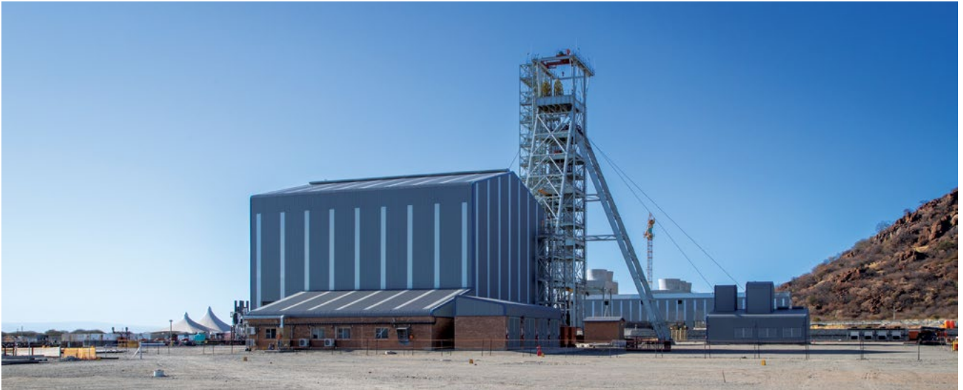
Zondereinde Western Expansion Project 3 Shaft headgear and winder-house.
