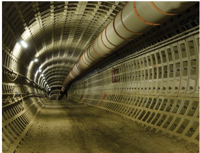
The Ghaghoo Sand Tunnel Project showing the concrete lined decline.
