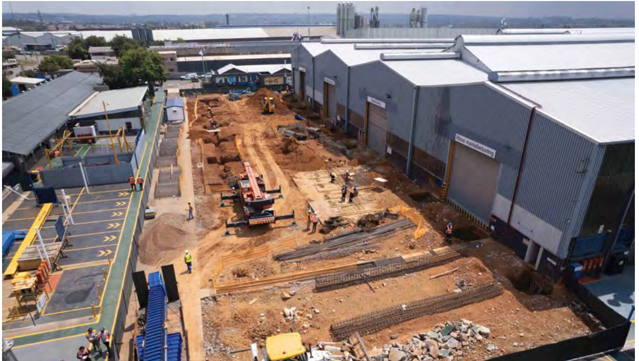
Construction of the new heavy bay screens manufacturing facility commenced in February 2025, with the project requiring substantial earthworks and piling to prepare the site for development.
