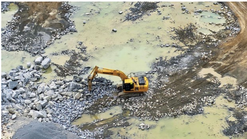
Secondary rock breaking plays a critical role at Rheebok Quarry to manage oversized blasted material and maintain efficient plant throughput.
