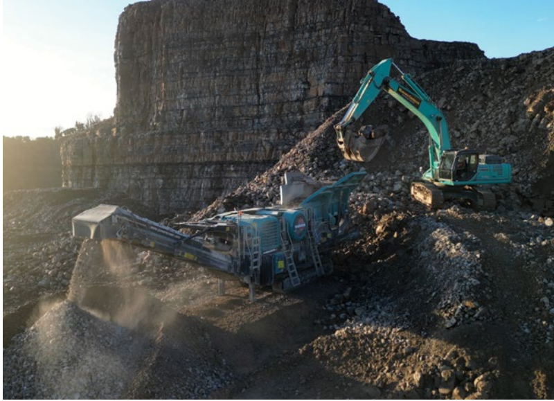
Conveyor maintenance can be dangerous even when LOTO and other safety measures are in place.
