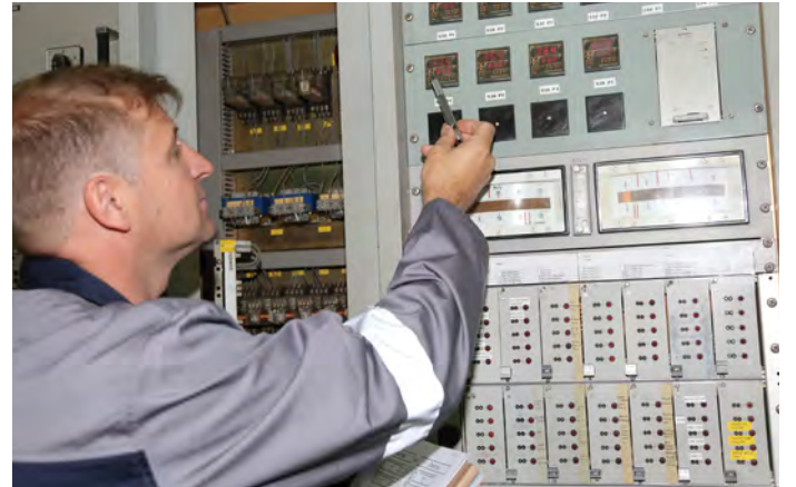
This safety circuit is required to undergo technical compliance testing every time a level one audit is scheduled. Here, testing is conducted by WearCheck advanced field services technician, Joe Kies, to ensure that it is operating within the required safety regulations. After each audit, WearCheck prepares a report containing all findings and the previous three audit results to establish performance trends.
