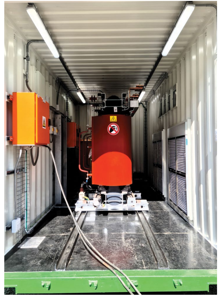
A 3 000kVA dry-type transformer fitted in one of the modular substations that is heading to the DRC's Bisie Mine.
